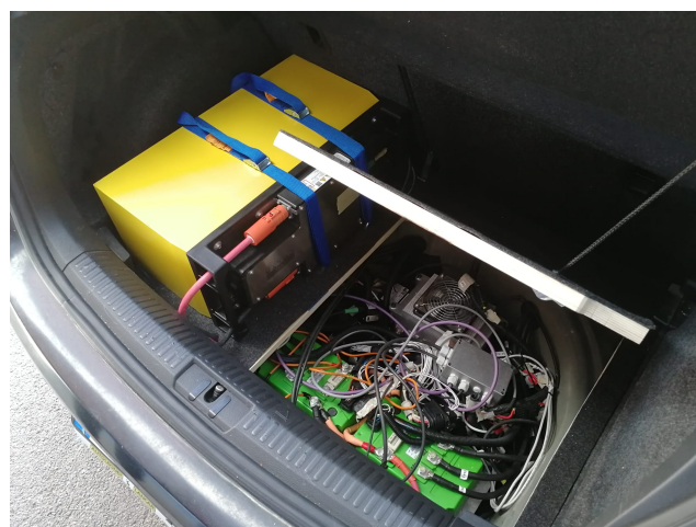
Fig. 6. Particulars of electronics in the VW Polo Prototype (Work in progress)
